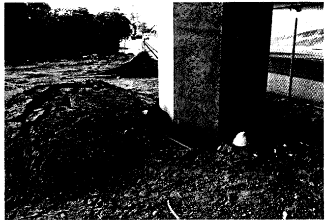
Fig. 10. Failure of column of I-10/Venice-La Cienega undercrossing.
